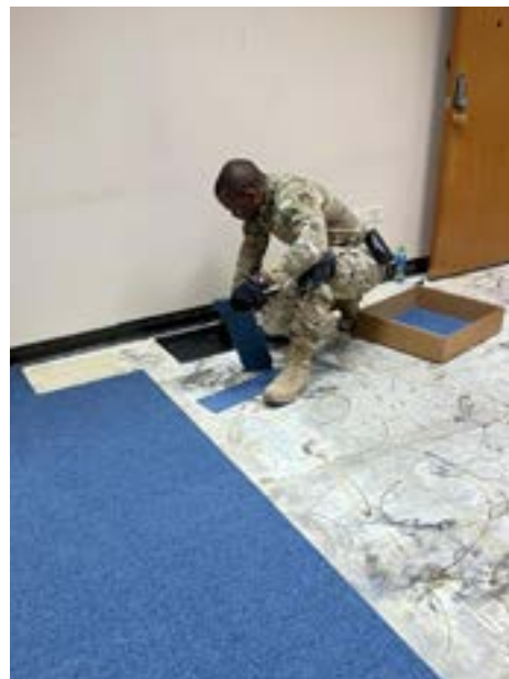
SrA Sylvain Nzeyang installing carpet flooring during a renovation project at Ali Al Salem Air Base. (courtesy photo)
